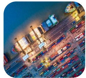
Dock, wharf, jetty
