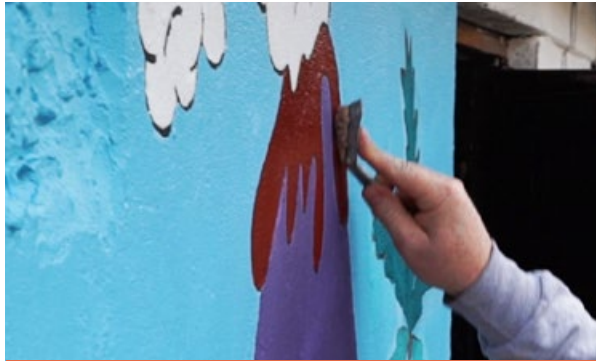
1. Cleaning and Prepping Wall
