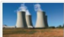
Accelerated Decommissioning Partners becomes licensed operator of Duke Energy's Crystal River Nuclear Plant
