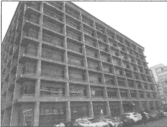
General view of the west elevation of the Site Building.
