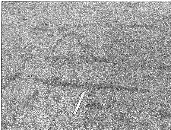
View of typical ridging in the BUR membrane.
