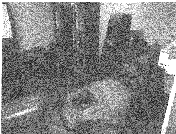
General view of within the elevator penthouse.
