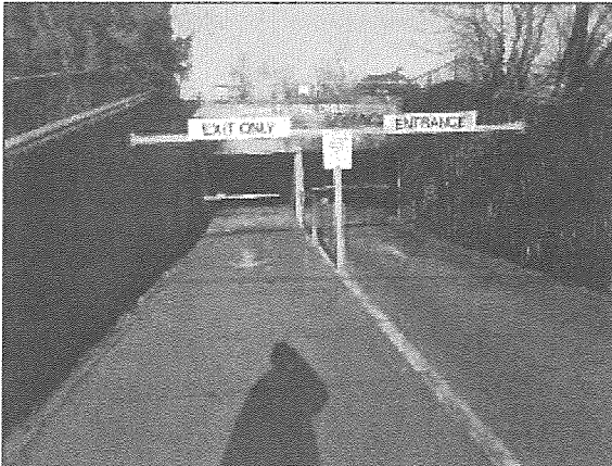
General view of the asphalt paved UPG ramp located on the south portion of the Site.
