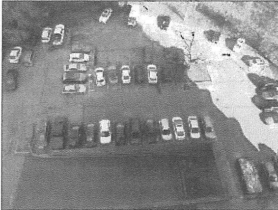
General view of the asphalt paved parking area located on the north portion of the Site.
